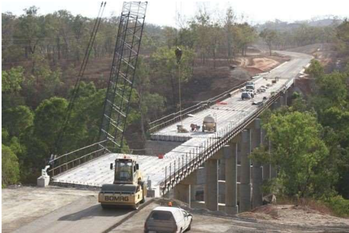
Building of the West Normanby River Bridge
