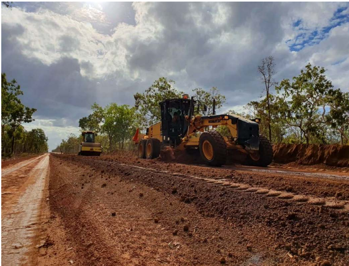
Aurukun Access Road – Bitumen Seal
